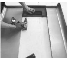
Fig. 43 - Secure the grate
