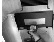
Fig. 30 - Secure the panel to the support
