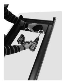
Fig. 23 - Secure the grate
