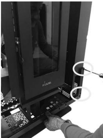
**Fig. 35 - Lower bracket fixing**
