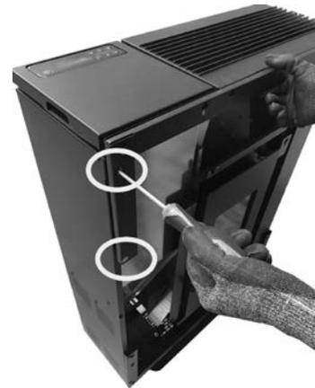
**Fig. 36 - Upper bracket fixing**
