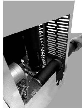
**Fig. 78 - Connect the ducting pipe**
