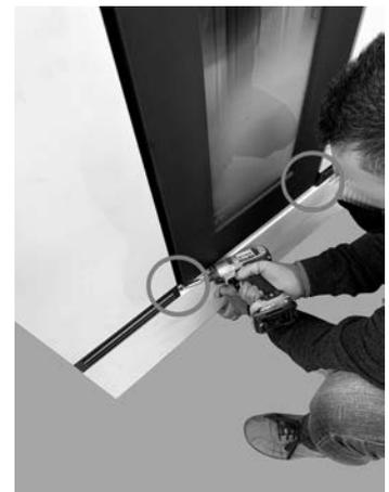
**Fig. 44 - Fix lower panel**
