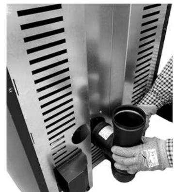
*Fig. 50 - Connect the Tee fitting*
