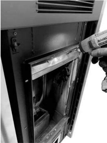
**Fig. 96 - Remove the deflector**
