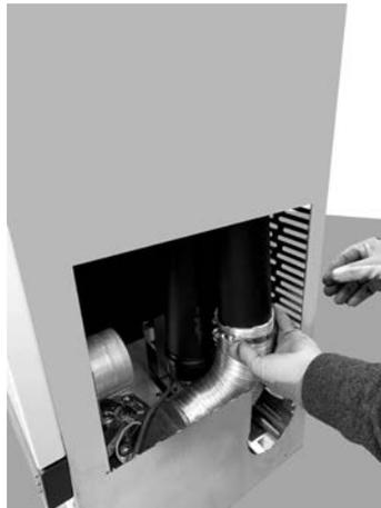
**Fig. 83 - Connect the pipes**
